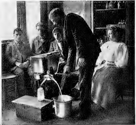
FIG. 220.—A modern hand separator. Cream separators of small size are used on dairy farms where cream or butter is sold.
